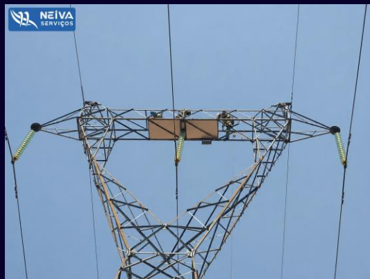
ANTI-PERCHING SYSTEM INSTALLATION (LIVE LINE)
